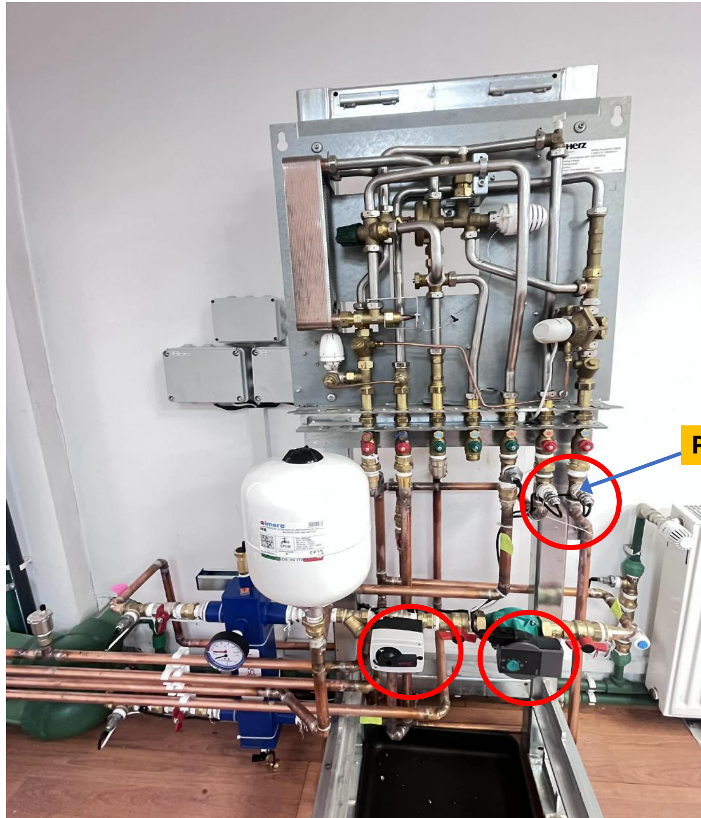
Heat interface unit (HIU) Three-way control valve Circulation pump and pressure equalization tank
